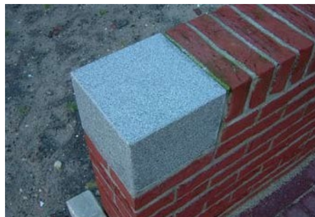
Quality low wall detail
