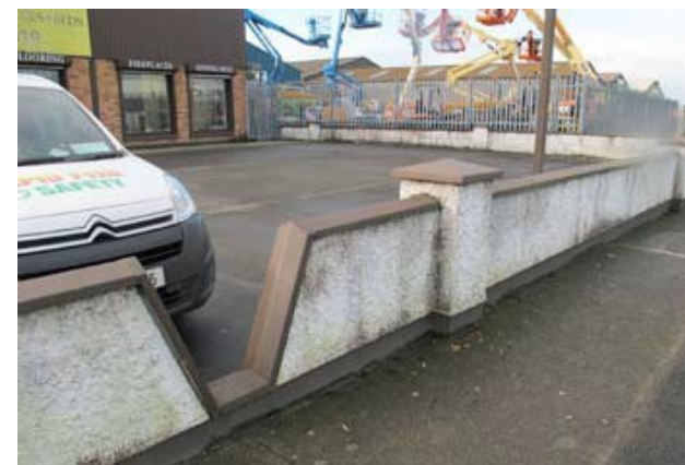
Pedestrian wall feature
