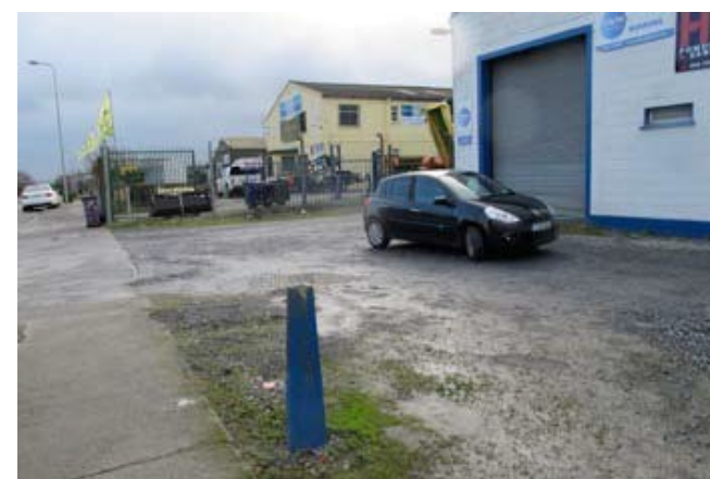
Poor quality frontage
