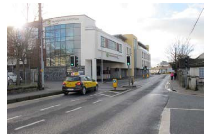
Basement car park entrance to Shopping Centre
