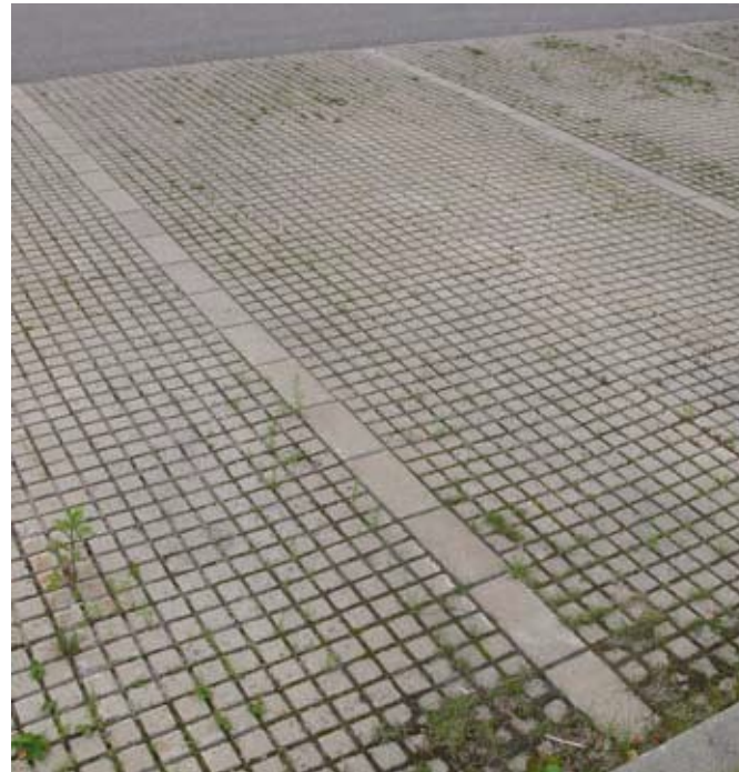
SUDS - permeable parking areas
