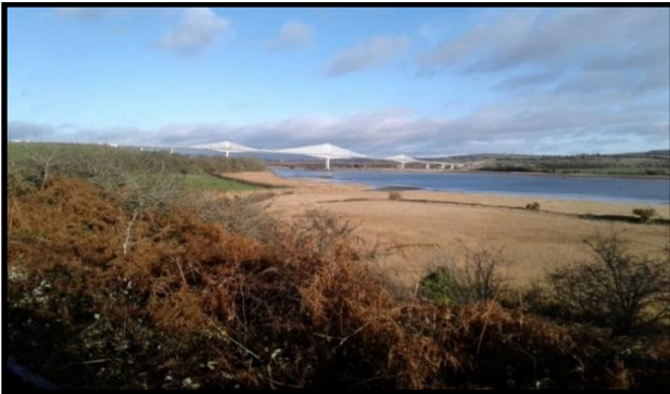
View from the Greenway towards the recently opened New Ross By-Pass bridge
