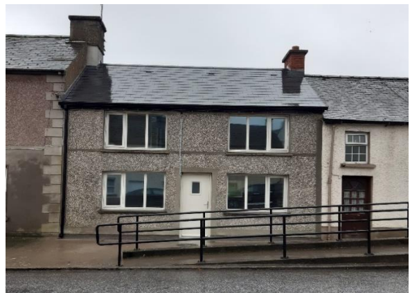
Refurbishment of 47 Barrack St, Castlecomer
