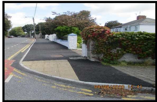
Footpath Works – College Road
