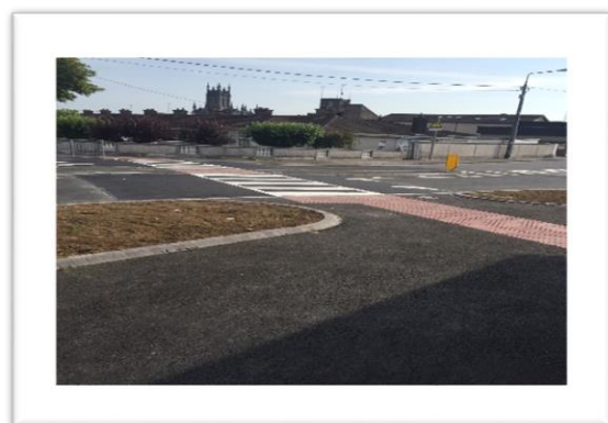
Gaol Road Junction Improvement
