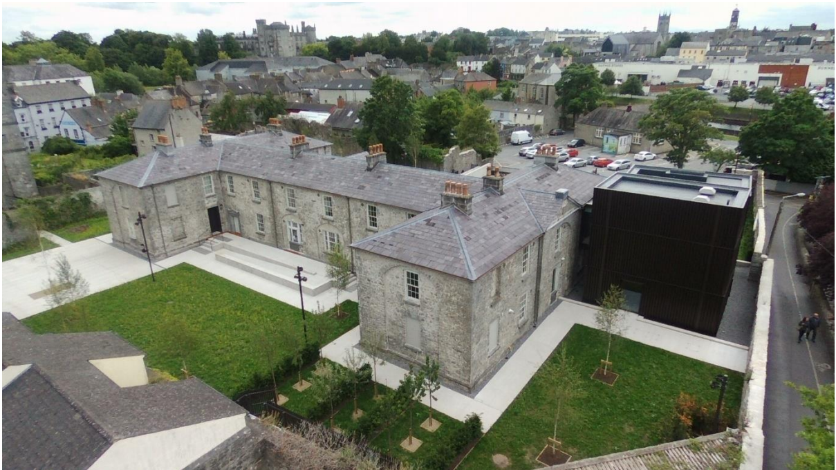
Rear of the building looking west with Kilkenny Castle, St. Mary Church & The Tholsel on the horizon
