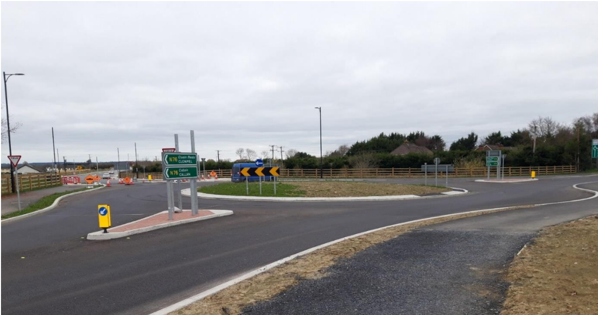
Kilkenny Western Environs Phase 1 Infrastructure
