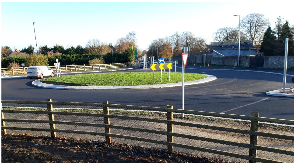
Kilkenny Western Environs Phase 1 Infrastructure
