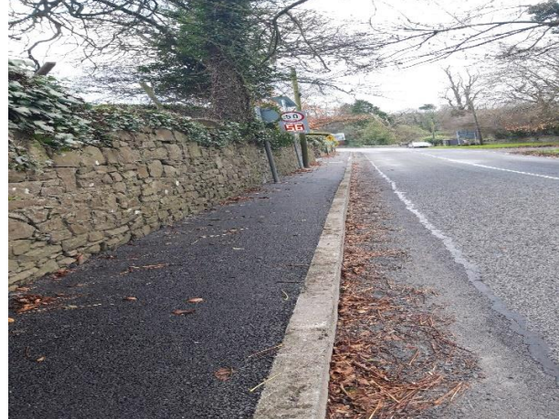
Footpath & Drainage, Clogh Road, Castlecomer
