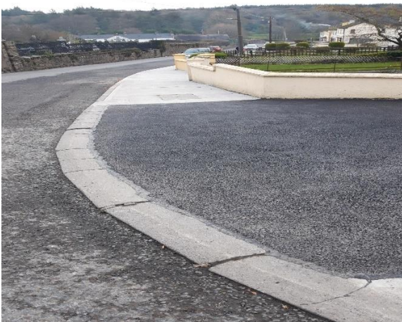
Footpaths at Maryville, Castlecomer
