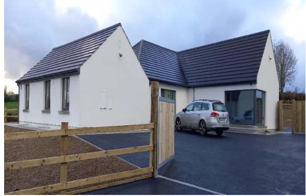
Group Home at Garraun, Windgap, Co.Kilkenny Good Shepherd AHB in conjunction with Kilkenny County Council
