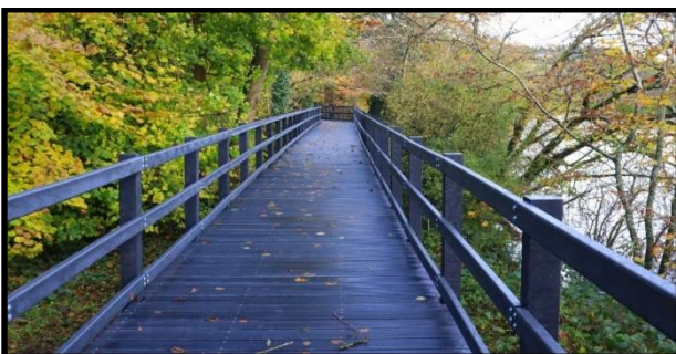
Silaire Wood Boardwalk Replacement
