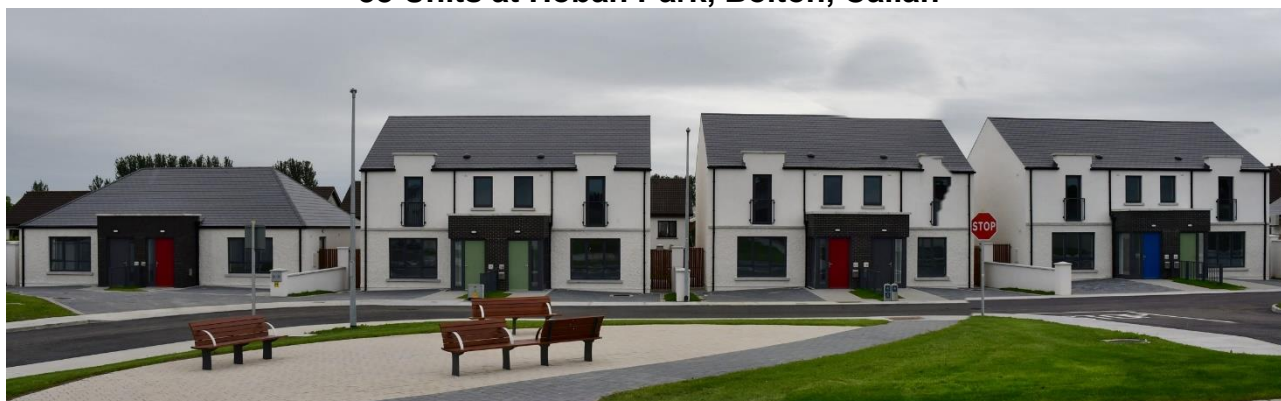
One of the first Nearly Zero Energy Building residential schemes built in Ireland A2 and A3 BER rating
