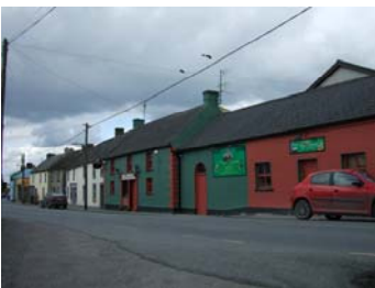
Poor road surface treatment
