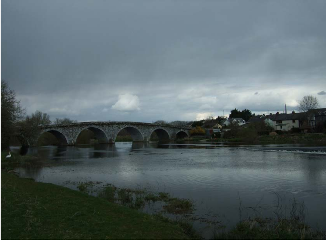
Figure 4: Looking northeast across river towards the bridge
