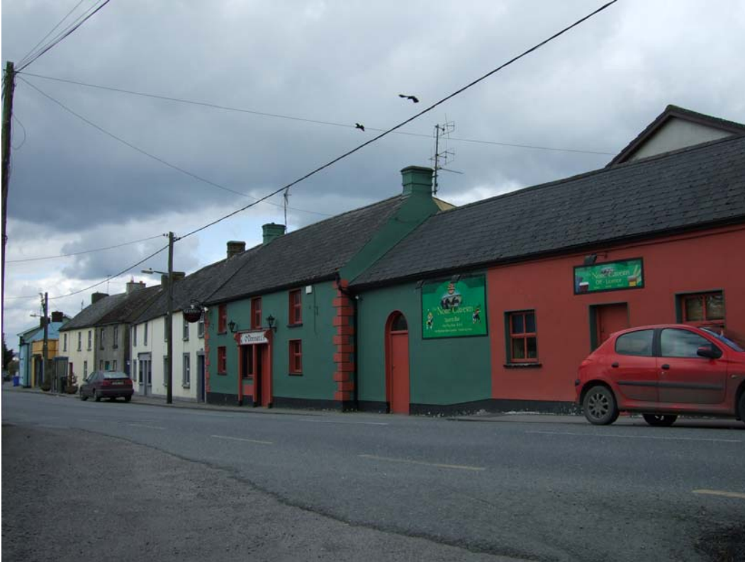
Figure 8: View of east side of Main Street showing buildings fronting directly onto the Main Street
