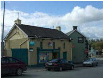
Main Shop in Bennettsbridge
