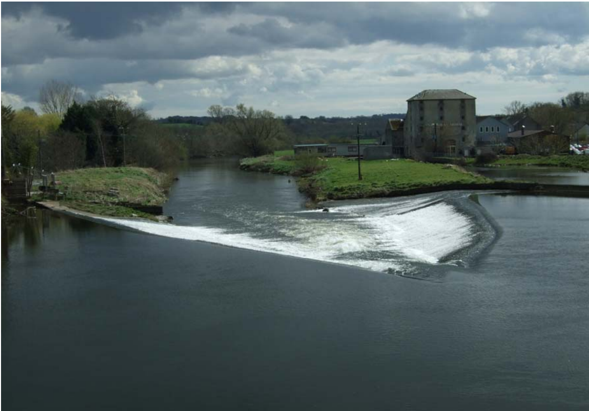
Figure 3: Mosse mill with weir to foreground
