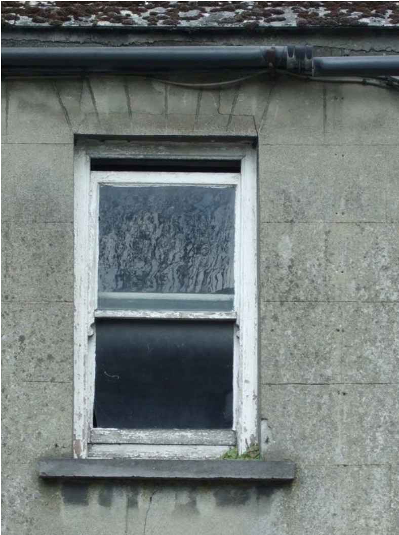
Figure 12: Examples such as multi-paned windows, most particularly the original sliding sash windows, of which few remain
