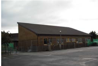
New School Extension
