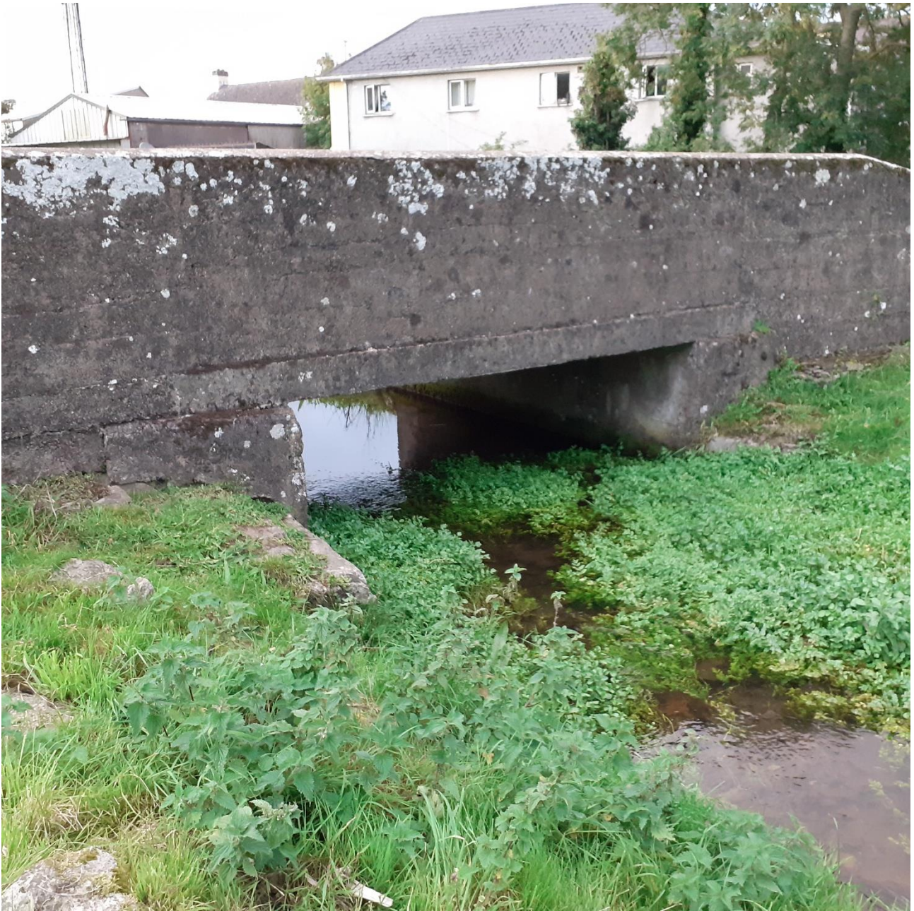
Plate 1: Bridge 10, Ballyhale, Co. Kilkenny.
