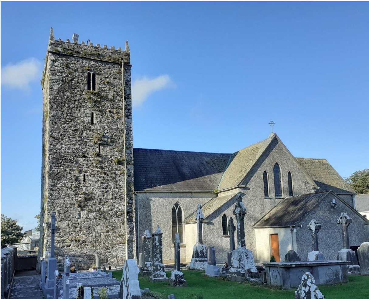
Plate 5: Church and tower, Ballyhale, Co. Kilkenny.
