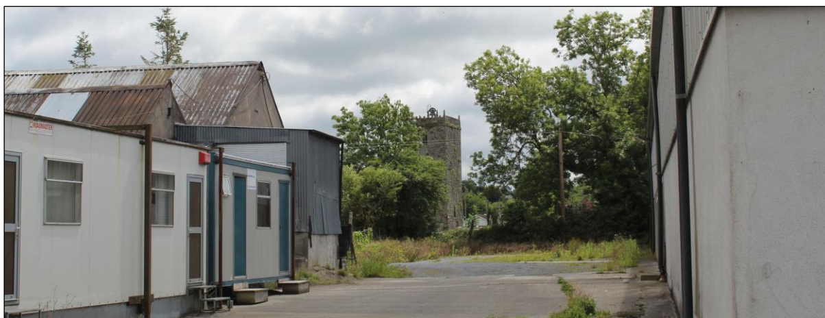
Plate 8-5: Stream is culverted under Arrigle business park
