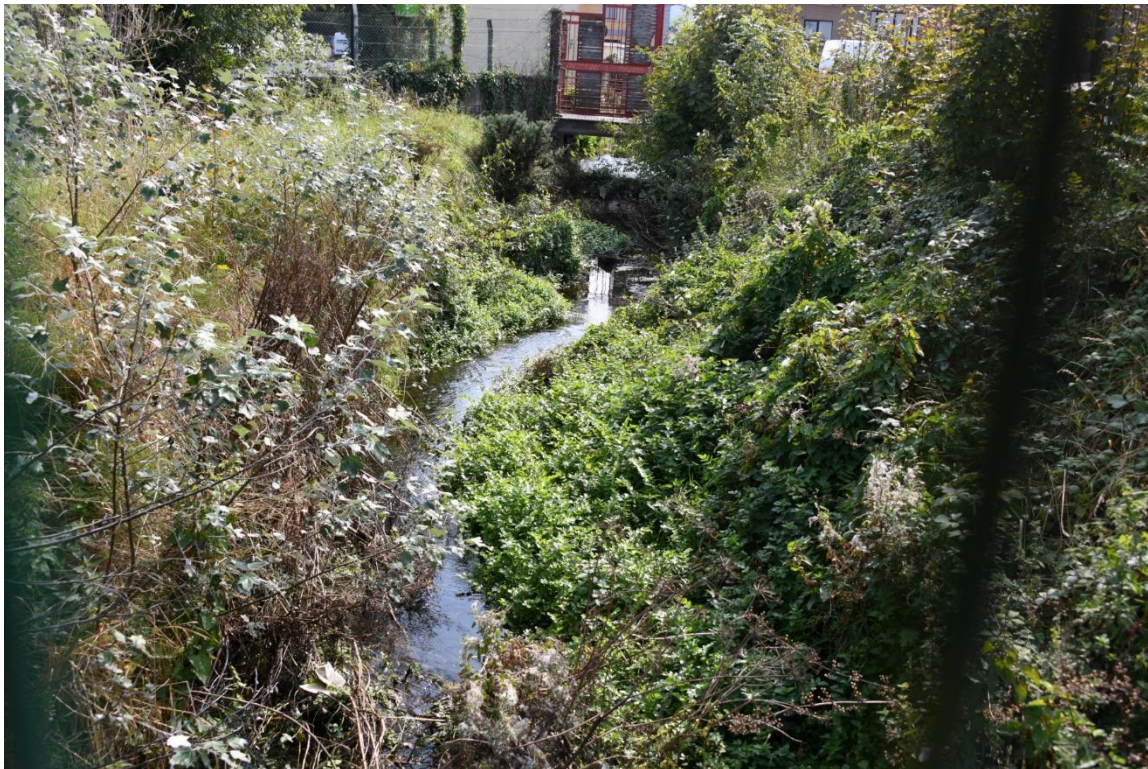
Plate 3. Bridge within the town with a 30cm high weir.
