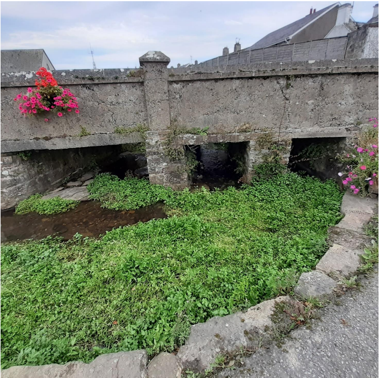
Plate 2: Bridge 8, Ballyhale, Co. Kilkenny.
