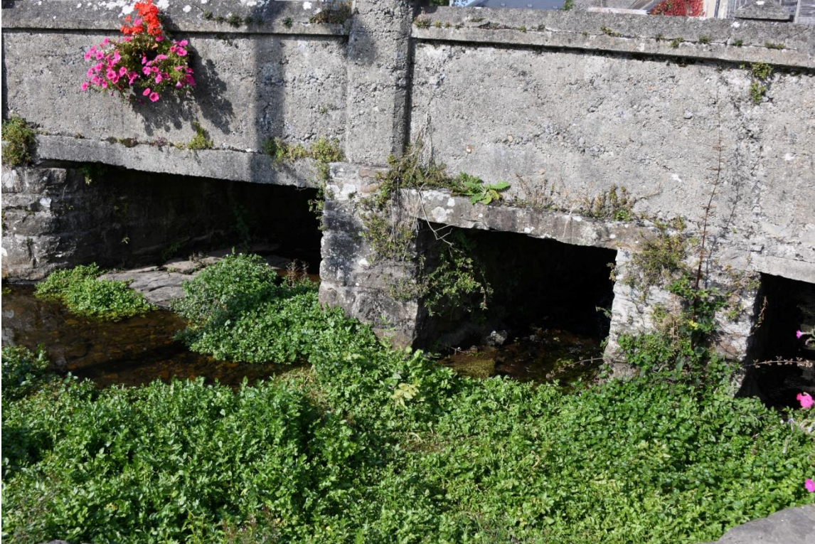
Plate 2. Bridge located at the downstream end of Section C
