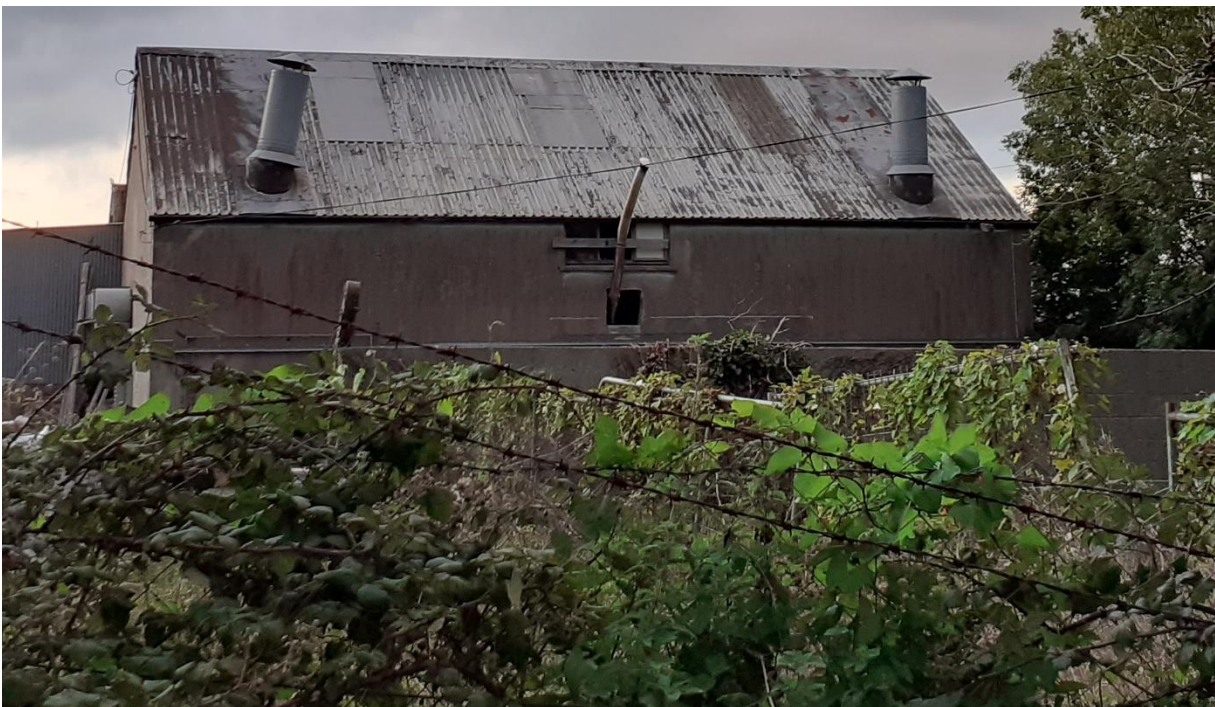
Plate 6: Shed, Ballyhale, Co. Kilkenny.
