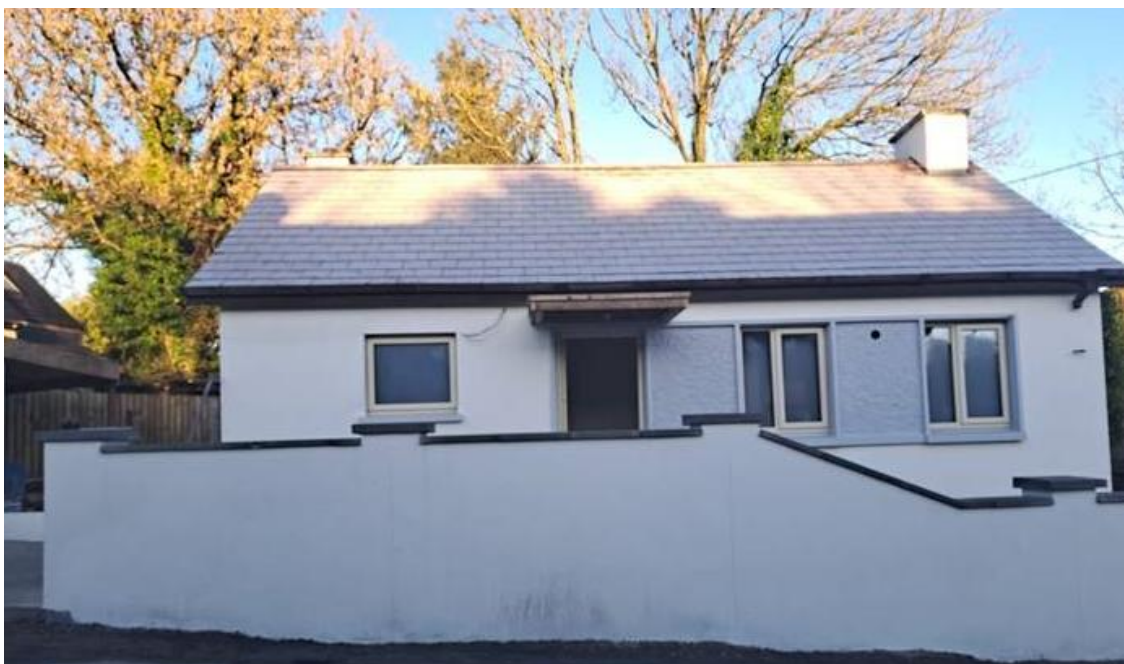
Conversion of the former Health Centre in Kilmacow to a 1 bed house is almost complete
