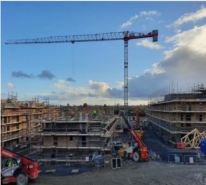
Crokers Hill, Kennyswell Road, Kilkenny City 88 Units due October 2024 – works ongoing
