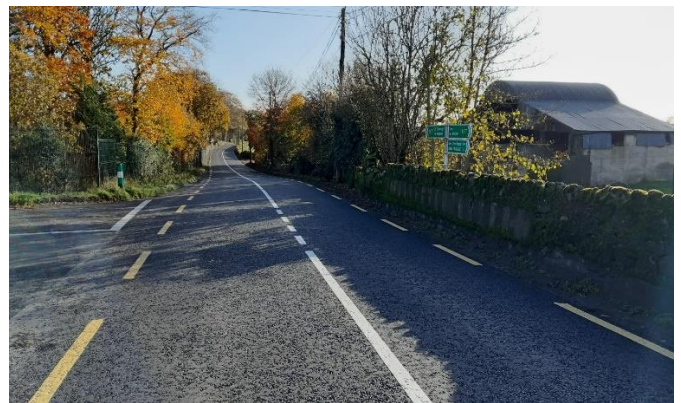
New pavement on the N77
