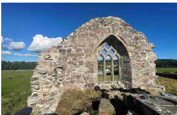
Conservation works at Thomple Church, funded under the CMF, 2023
