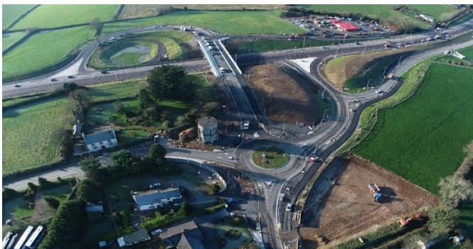
Overhead drone footage of the compacted grade separated junction under construction.
