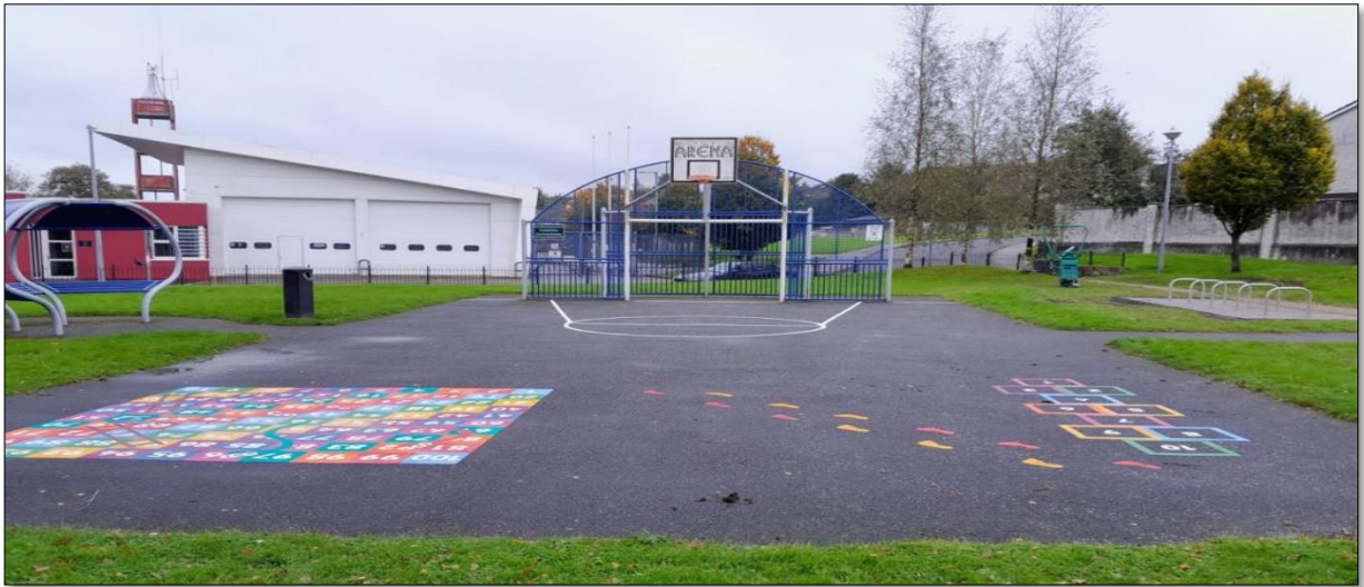
Enhancement Works completed in Castlecomer MUGA
